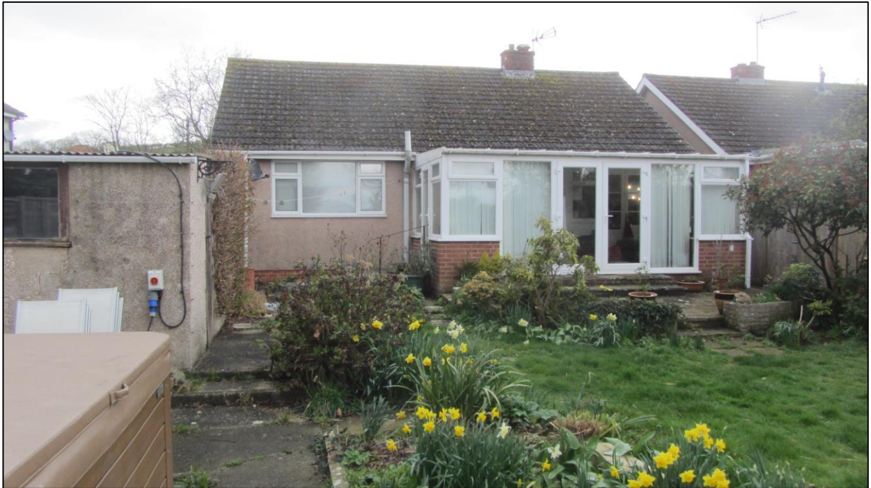
Plate 1. View looking NE showing rear of property with existing extension.
